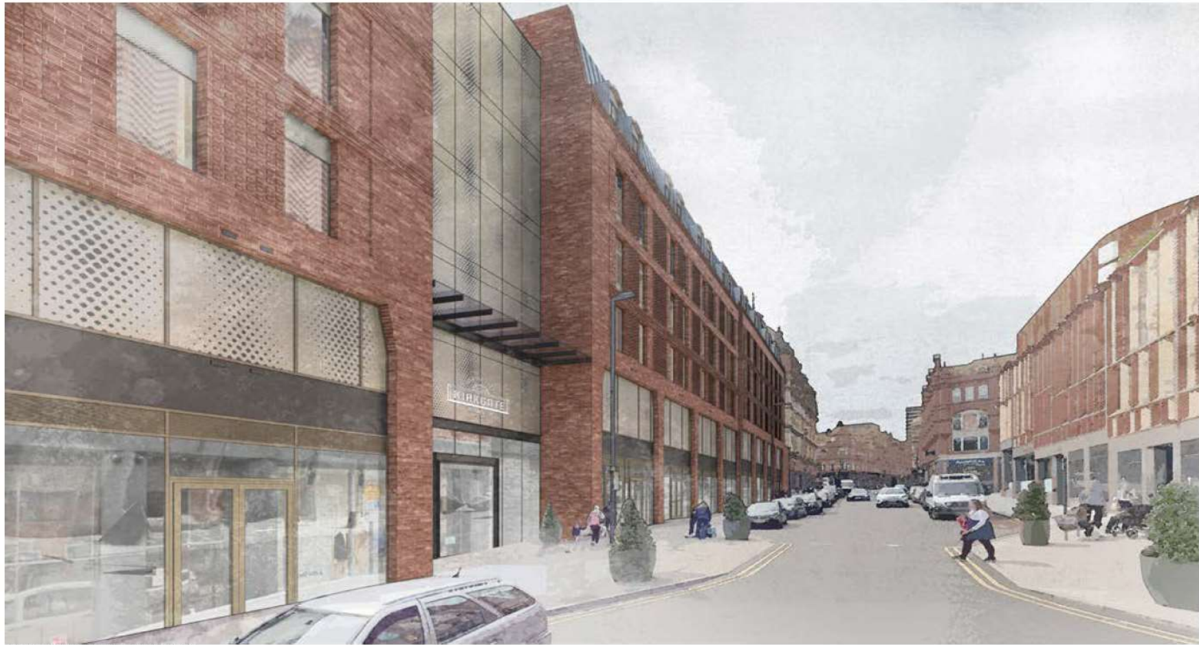
View West along George Street
